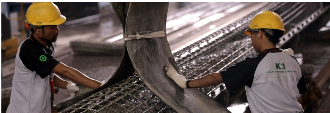
Gambar (Illustration) 04. Proses Pengecoran/ Pouring Concrete
