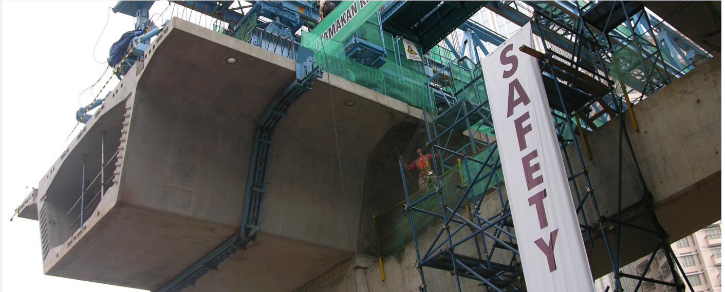
Gambar (Illustration) 14. Instalasi Box Girder proyek Bogor Outer Ring Road /Box Girder instalation at Bogor Outer Ring Road
