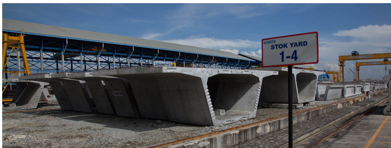
Gambar (Illustration) 15. Persediaan Box Girder/ Box Girder stock
